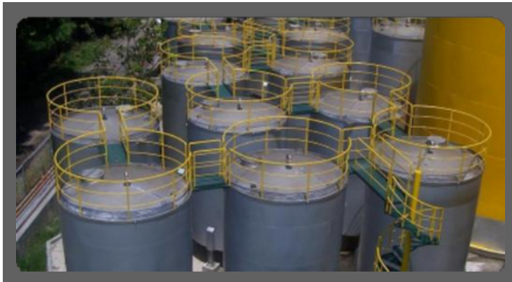
Fabrication / Installation of 16-Unit 30 Tons SS Tank
