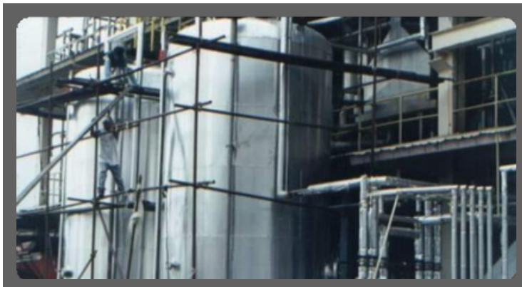
Fabrication/Installation of Buffer Tanks, Pipe Works, Insulation
