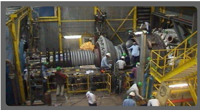
CCGT MAJOR OUTAGE
