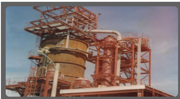
Fabrication / Installation of Acid Regeneration Plant
