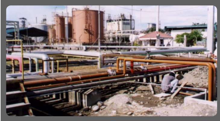
Installation of Waste Water treatment Plant Equipment
