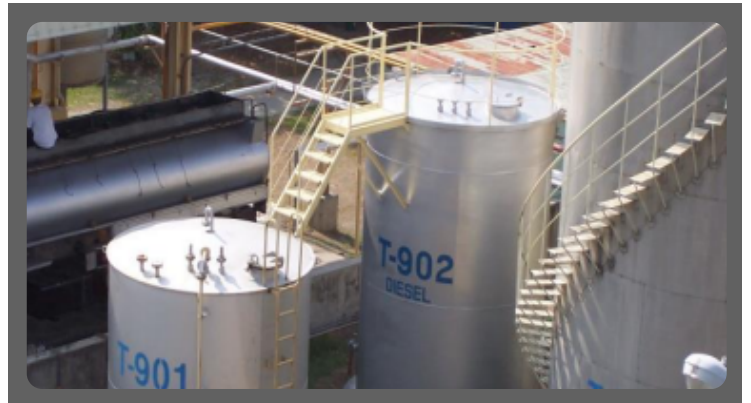
Fabrication / Installation of Diesel Storage Tank
