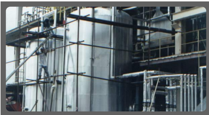
Fabrication/Installation of Buffer Tanks, Pipe Works, Insulation
