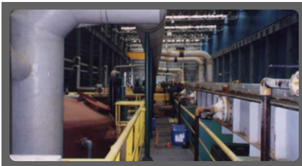
Fabrication / Installation of Pickle Tank
