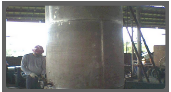
Fabrication / Erection of T-863
