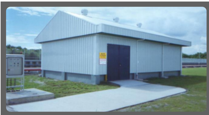
WASTE STORAGE BLDG
