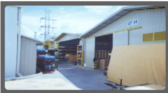
RESTORATION OF WAREHOUSE
