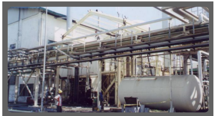
Fabrication/Installation of Boiler Roof structure, Storage Tank and Thermal Heater
