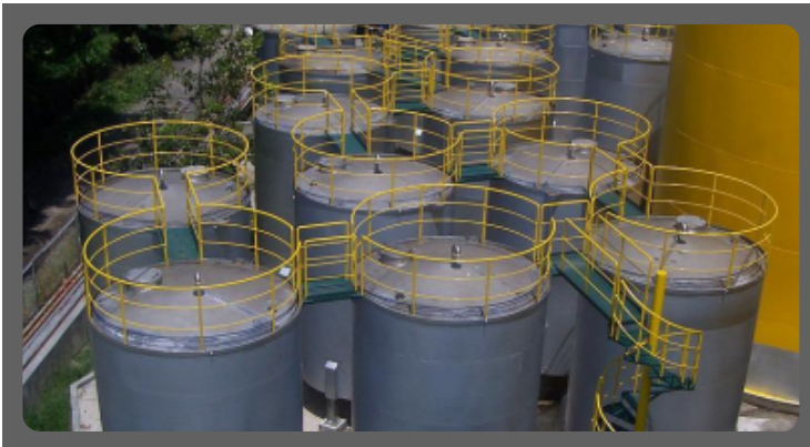
Fabrication / Installation of 16-Unit 30 Tons SS Tank
