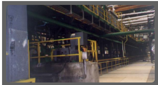
Installation of Electric Furnace and Piping
