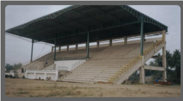
Fabrication / Erection of PSC Grandstand
