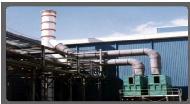
Fabrication / Erection of Exhaust Fume Stack
