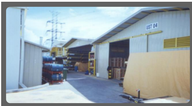
GLOBAL MARINE BLDG Balete, Bauan, Batangas
