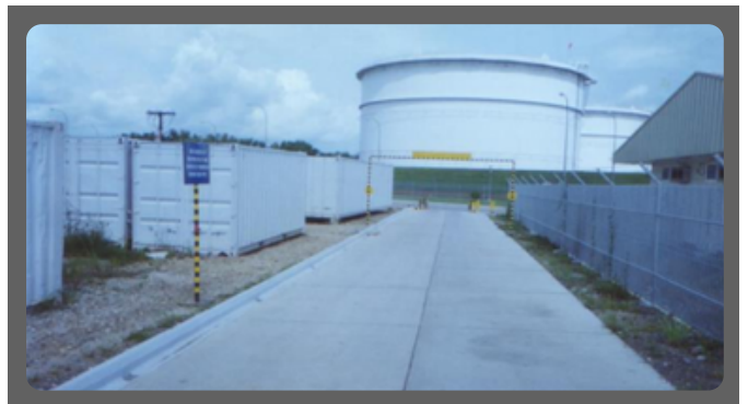
ADDITIONAL ROAD AND BRIDGES
