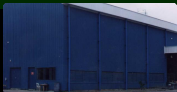
Construction of General Store
