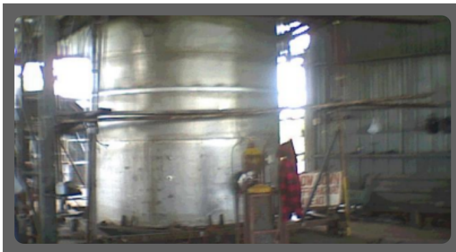
Fabrication / Erection of Tank T-862
