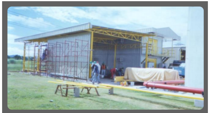
ELEVATED CONTAINER CANOPY
